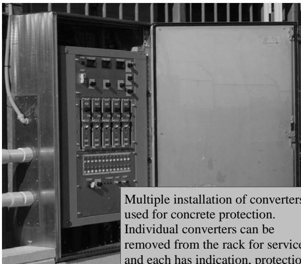
Multiple installation of converters used for concrete protection. Individual converters can be removed from the rack for service and each has indication, protection and output control.
